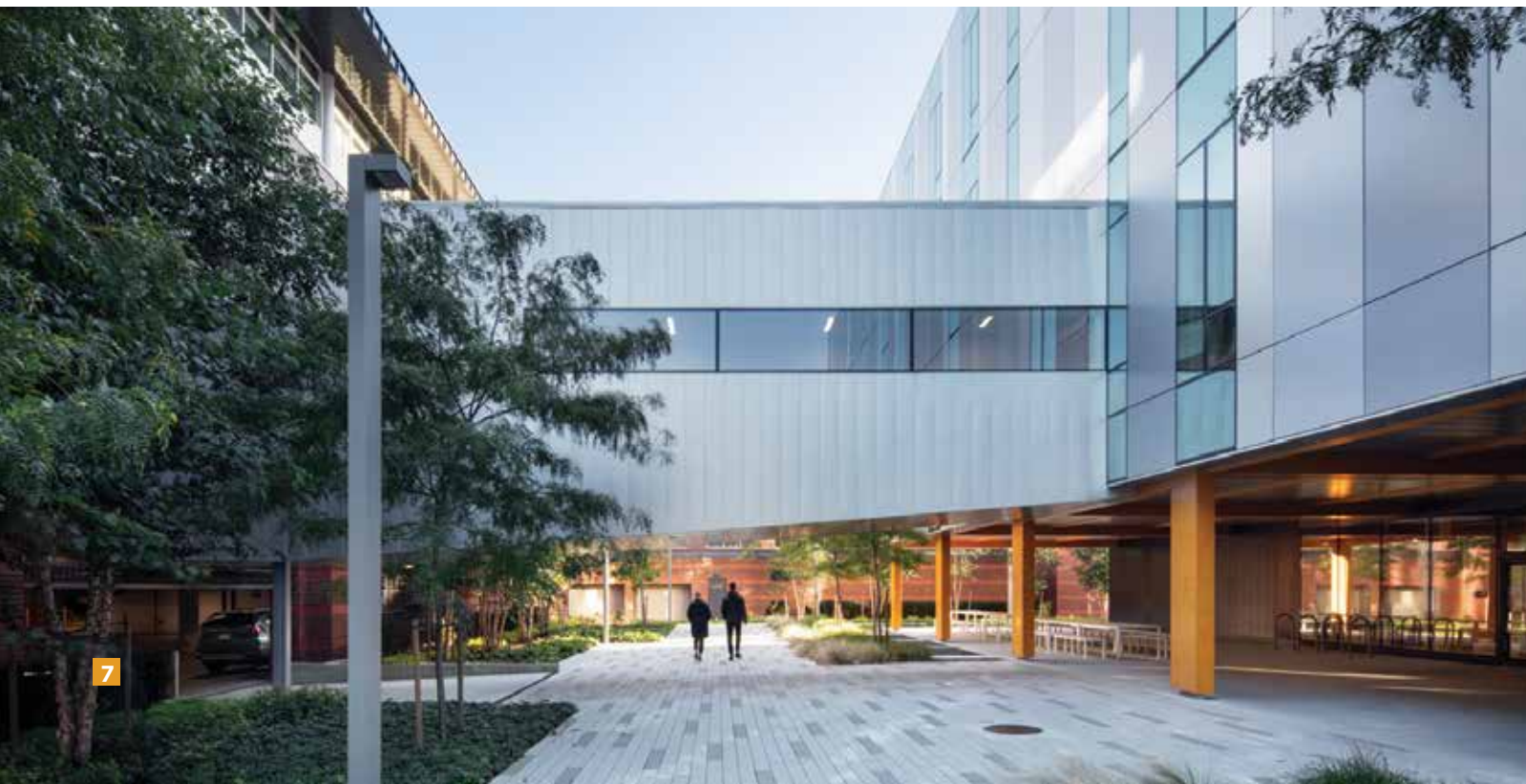
7. The connecting bridge extending from the east elevation.
